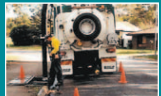
Specialised services: hydro-excavation/non-destructive pot-holing, confined space specialists.
