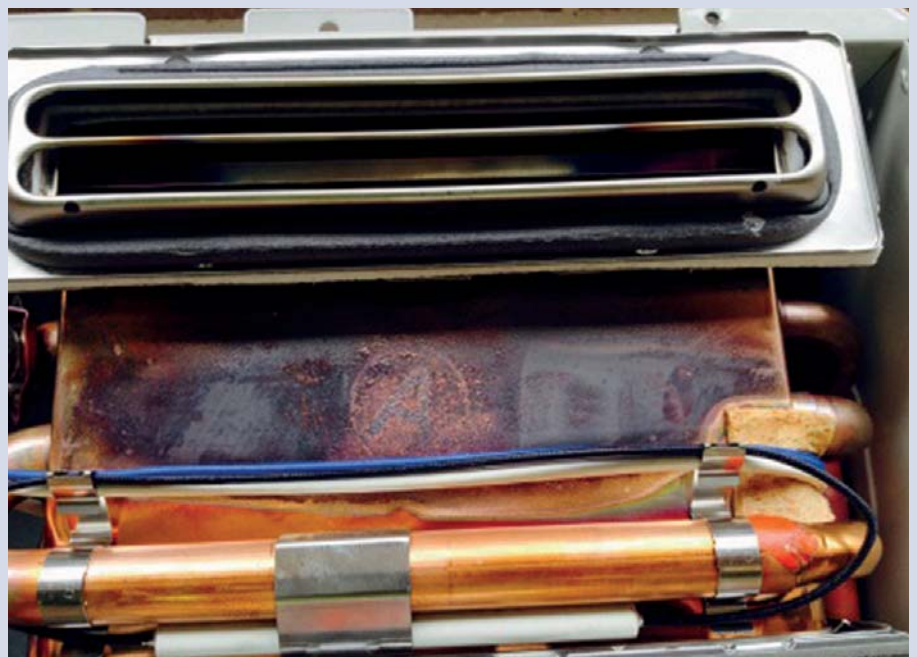
A hot water heater exposed to an excessive inlet operating pressure, required a two-week old unit to be replaced.
