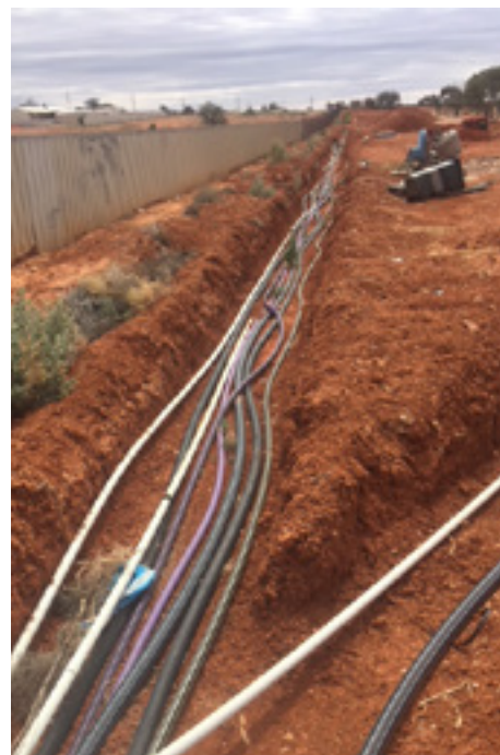
Underground services without correct separation.
