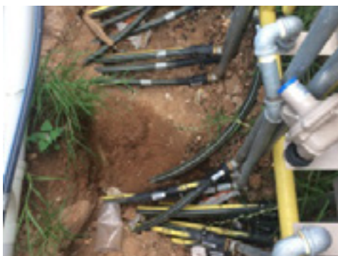
Examples of non-compliant installations (what a mess!)
