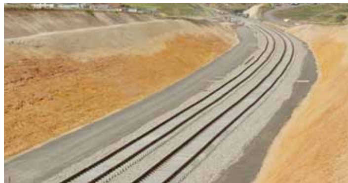
Above: Track extension from Noarlunga Centre towards Seaford.
