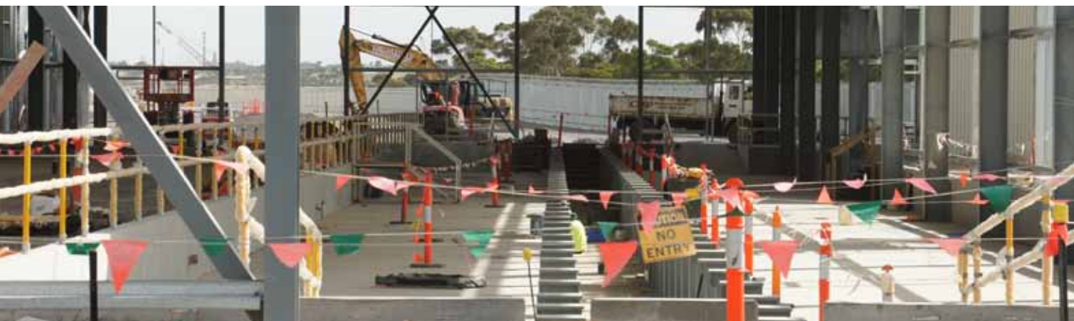
Above: General maintenance shed under construction at the Seaford Rail Yard.
