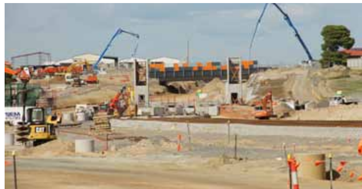
Above: Seaford Road bridge under construction.
