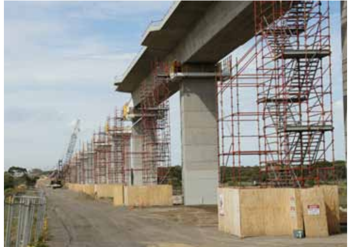
Above: Onkaparinga Valley Bridge under construction.
