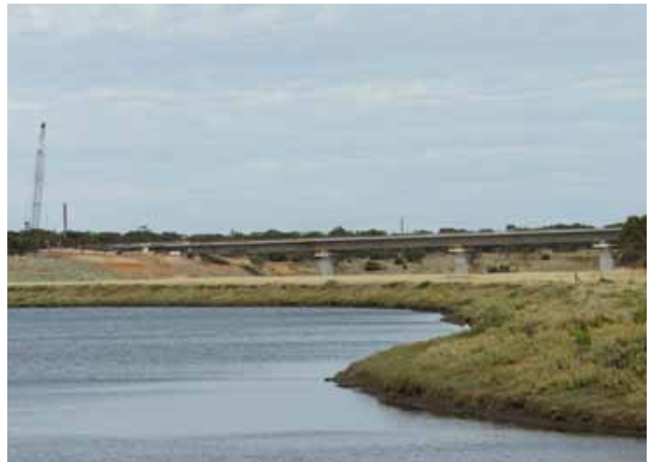
Above: A section of the Onkaparinga Valley Bridge nearing completion.
