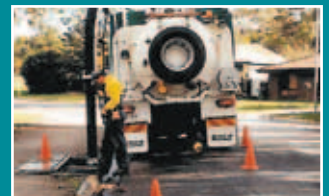
Specialised services: hydro-excavation/non-destructive pot-holing, confined space specialists.
