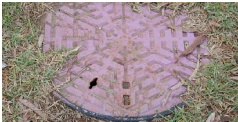
Above: GAP Recycled water valve box cover
