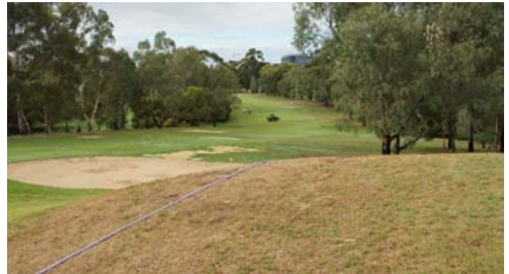
Above: North Adelaide Golf Links with GAP Recycled water purple pipe on one of the tees
