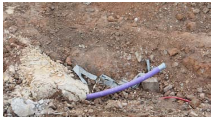
Above: New recycled water pipe in Victoria Park
