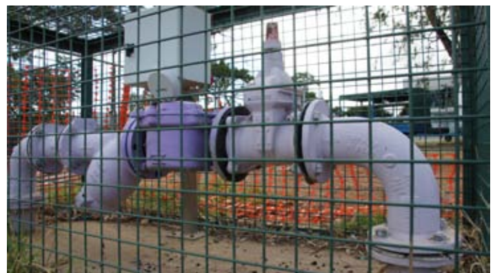
Above: GAP Recycled main valve station
