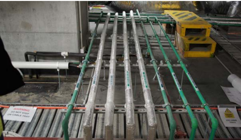
Above: Domestic Hot Water and Laboratory water pipe work
