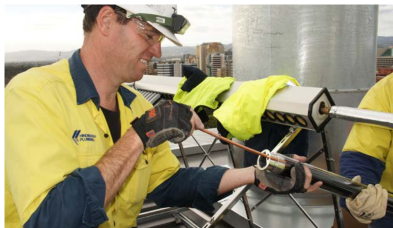
Above: Chris Day (2nd year apprentice) installing evacuating tubes on the roof
