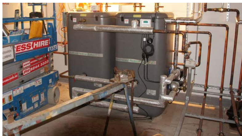
Below: Rotex heat exchangers in the Plant Room
