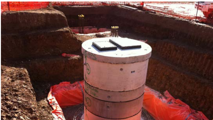
Above: Stormwater pump station
