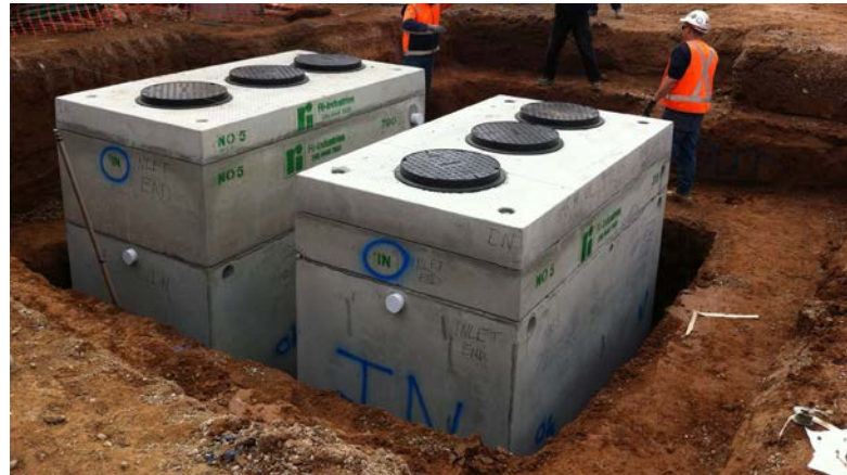
Above: Grease arrestors with a Mag Flow meter being dropped in
