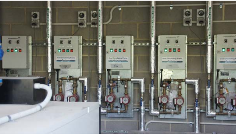
Above: Fresh water circulating pumps
