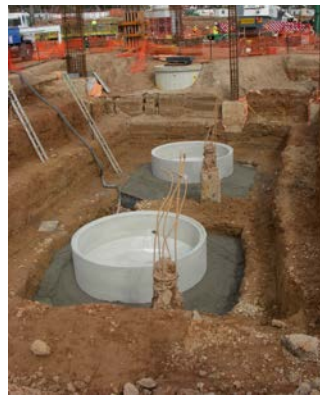
Above: Sewer pump stations
