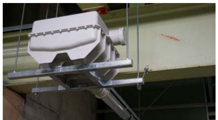
Above: Demonstration "Drainwave Unit" installed within the Plumbing Rig.
