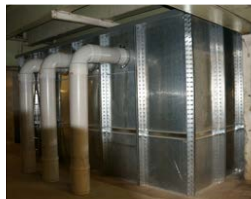
Above: 700kl Rainwater Recycling Tank
