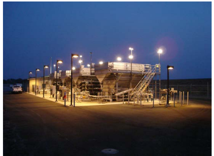
Above: Nijhuis DAF plant at night
