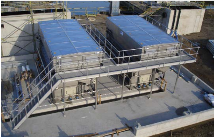
Above: Nijhuis DAF plant
