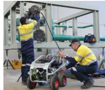
Above: Peter Orr and Ramy Saleed of Adept Engineering, Chatswood use an Aussie hydrotester to test the integrity of desalination plant modules before they are transported to site.
