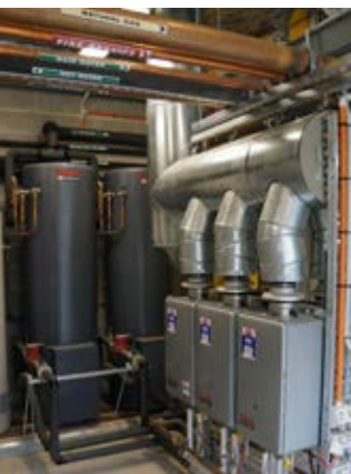
Above: Hydraulic Plant Room
