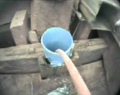
Above: Exposed Downpipe
