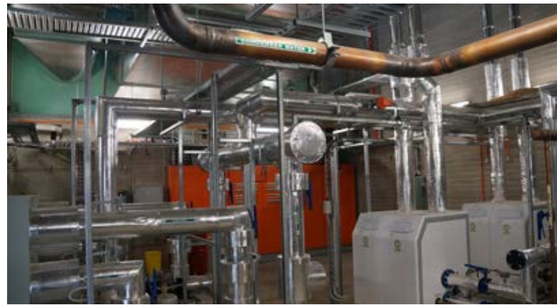
Above: Mechanical Plant Room
