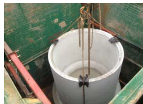
Above: Sewerage Ejection Pump Station
