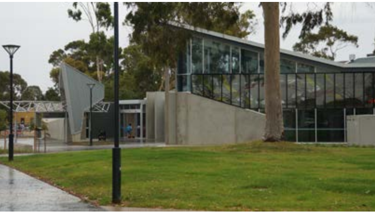
Above: Parks Community Centre
