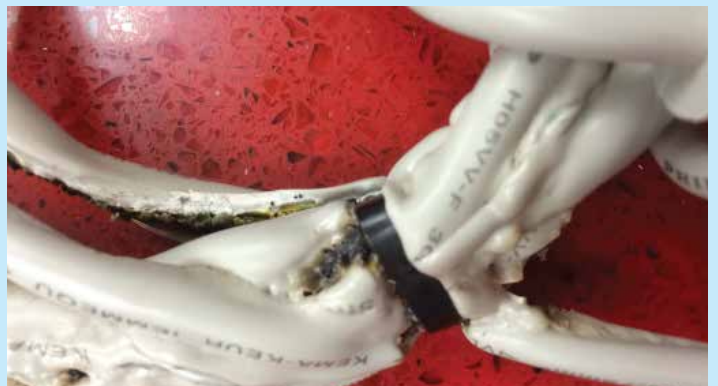
Above: Cable Tie Creating Electrical Fire Risk
