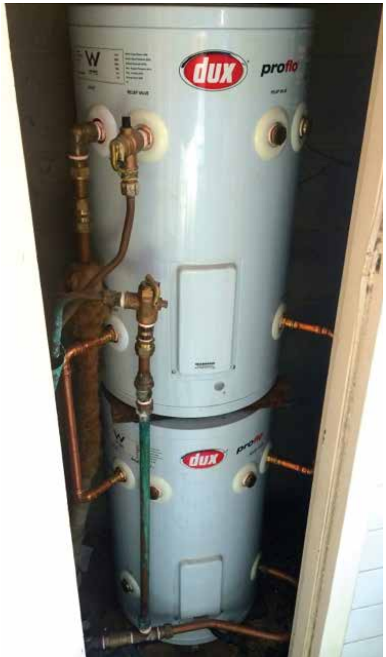
Above: An inappropriate solution to a problem
