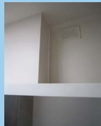
Above: Pipe work runs along the inside of the room instead of being concealed
