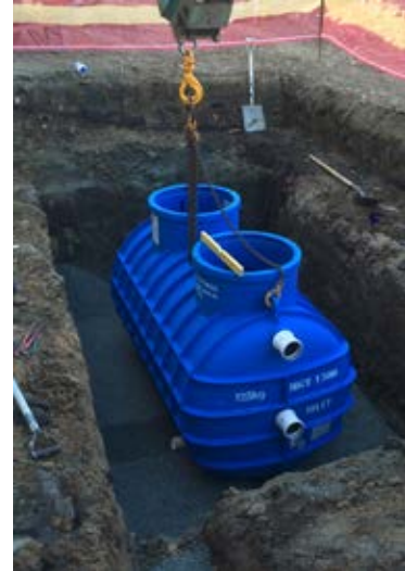
Above: Woolworths Aberglasslyn Crane
