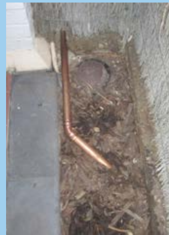
Above: Copper pipe laid on ground
