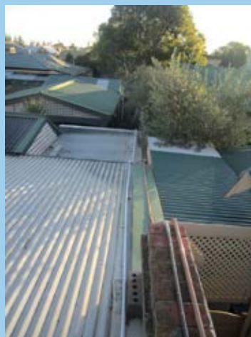
Above: Copper pipe pipe running along the top of the common wall
