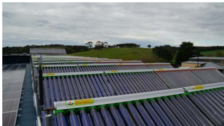
Above: 960 tubes making up the array.
