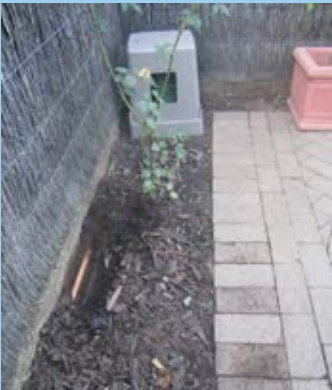
Above: Copper pipe laid on ground
