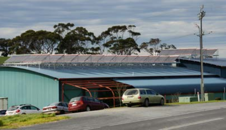
Above: Paris Creek factory with roof top tube array.
