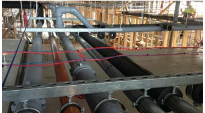
Above: Instaflex & copper mains reticulation
