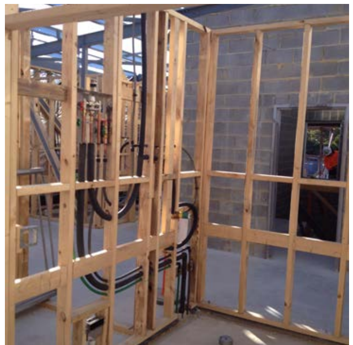
Above:Typical ensuite - Rehau inwall pipework, Enware TMV and Blucher Tundish
