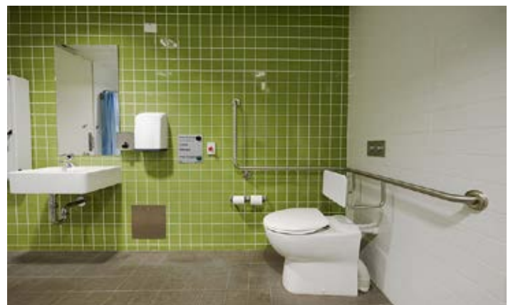
Above: Accessible sanitary facilities in buildings covered by the code must be installed according to AS 1428.1 2009.
