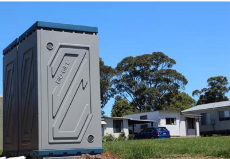
Above: BioGill bioreactors treating wastewater onsite at Tomago, near Newcastle.
