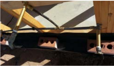
Above: Incompatible PE fittings / pipe components.
