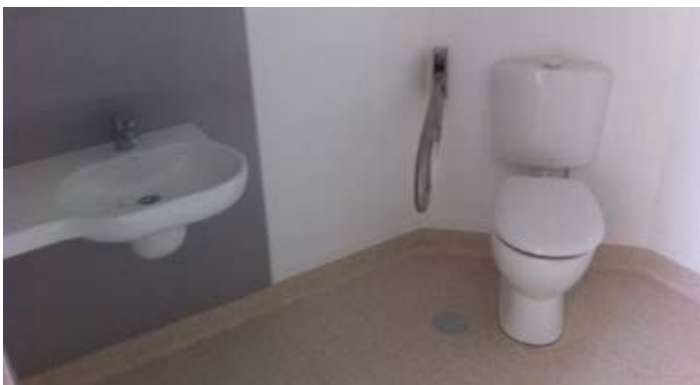
Above: Typical ensuite installation
