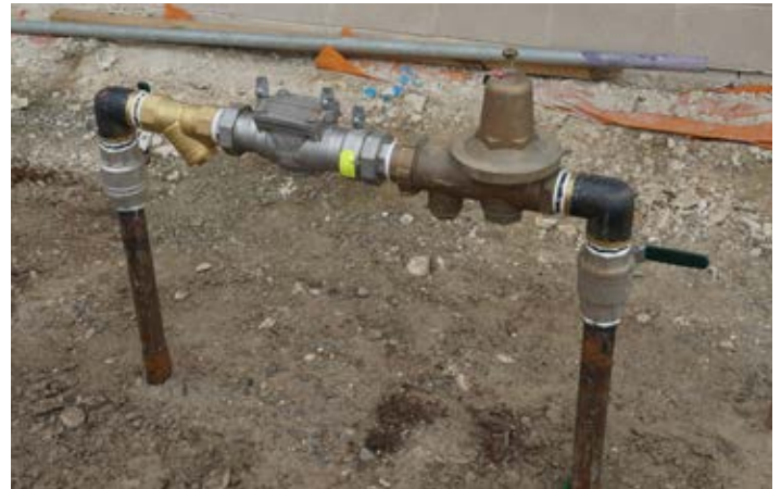
Above: Line strainer double check valve assembly and pressure reduction valve
