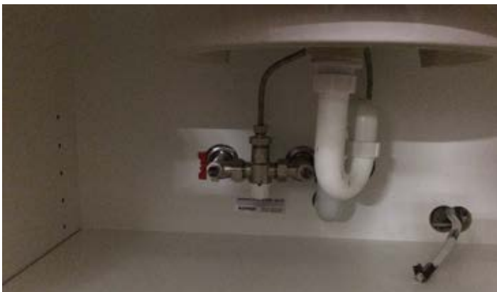
Above:TMV under sink in cupboard
