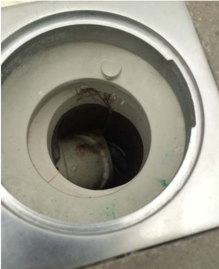
Above: A very poorly installed and misaligned shower grate on an 80mm riser pipe simply drilled and silicone used to allow a bath connection via 40mm being pushed in, what were they thinking?
