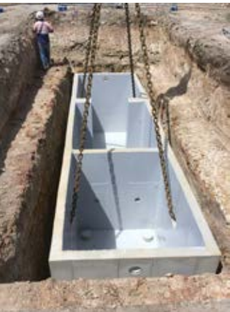
Above: 30,000 litre septic tank
