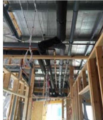
Above: Instaflex & copper mains reticulation
