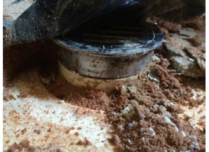
Above: A short chrome grate that has been installed with a butt connection pipe piece to reach the puddle flange which caused significant water damage to a property in inner Adelaide, as you can see the screed is damp.
