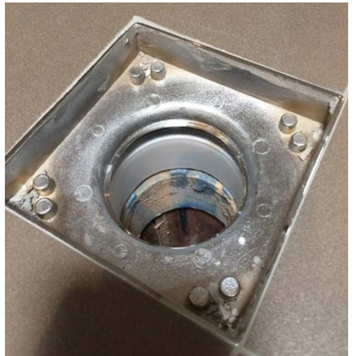
Above: This is an example of a job he has just completed for a client in the eastern suburbs with a smart grate. (Remember the white spacer seen here is socketed with the smart grate going into it). Repair success rate 100%.
