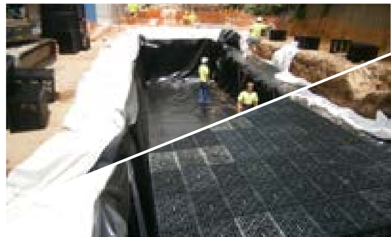
Above: Underground retention tank under construction
