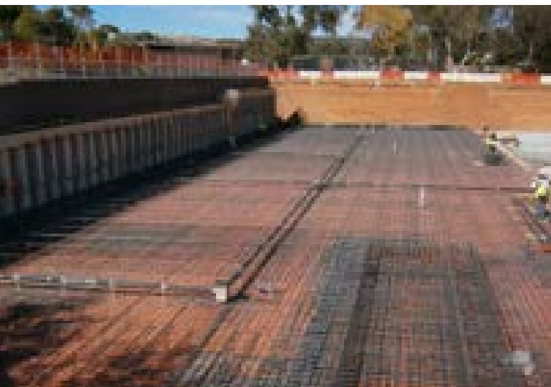
Above: PVC stormwater drain suspended within the slab
