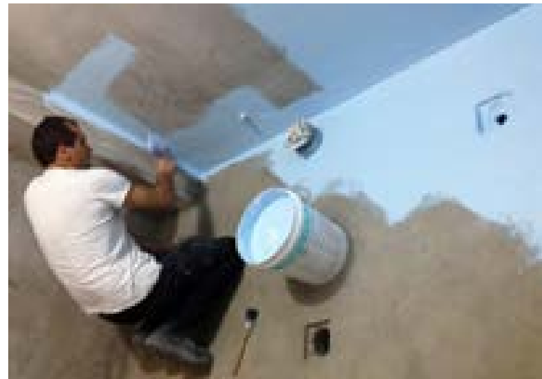
Above: Tiler waterproofing a bathroom
