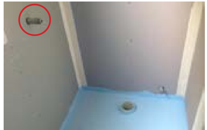
Figure 4: Example of a water connection point installed in a toilet room adjacent to a toilet.
