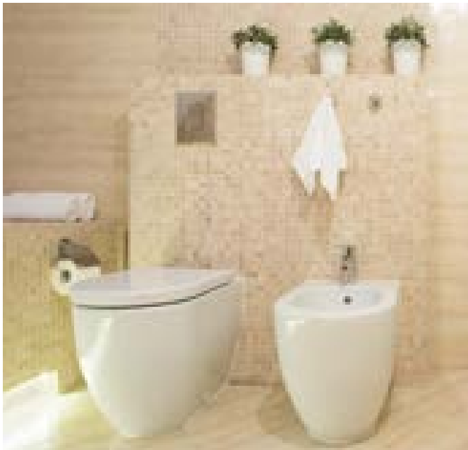
Figure 5: Example of a bidet with an outlet more than 25mm above the rim of the fixture.
