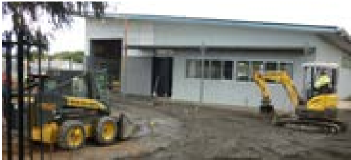
Above: Unley High School Skills Centre under construction
