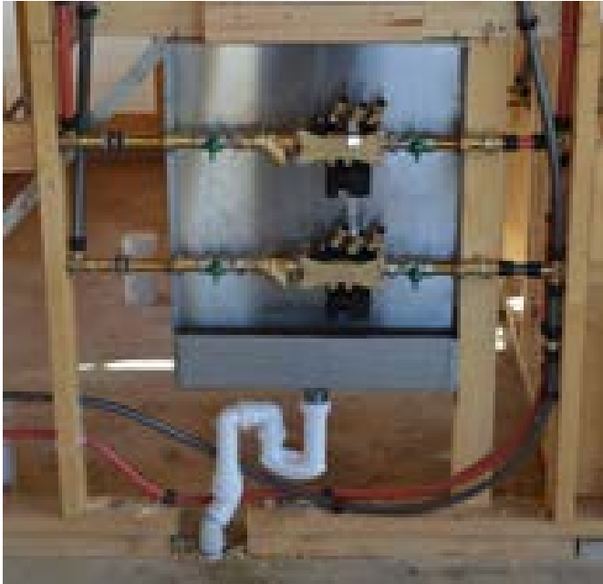
Figure 1: Example of 20mm reduced pressure zone (RPZ) device valve assemblies installed upstream of a flexi-spray outlet in a domestic setting.
