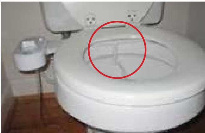
Figure 3: Example of a toilet seat douche outlet below the rim of the pan
